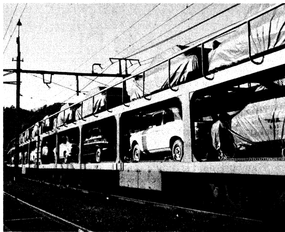
Figure 6: Japanese double-deck car, especially designed for carrying automobiles; it can load up to 12 compact cars.
